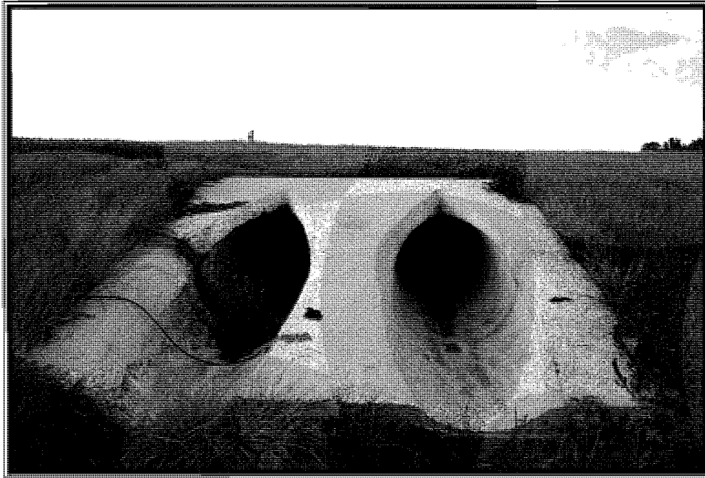
Photo 3-1. Culverts at OCF. These culverts are free of vegetation that could potentially impede water flow. Water is allowed to move quickly and easily through these culverts to properly drain the AOA.
